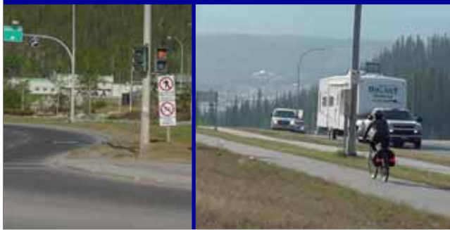
Bike path only on one side – numerous crossings from the wrong direction
