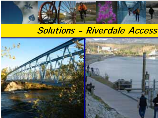
New pedestrian bridge
