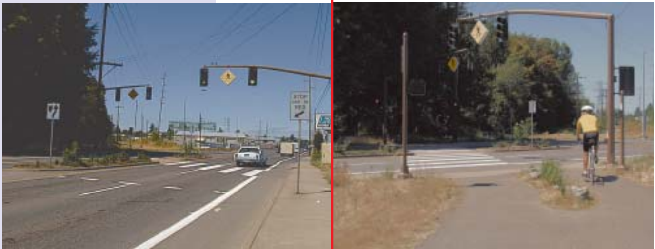
Trail crossing of highway with signal, median and high-visibility crosswalk
