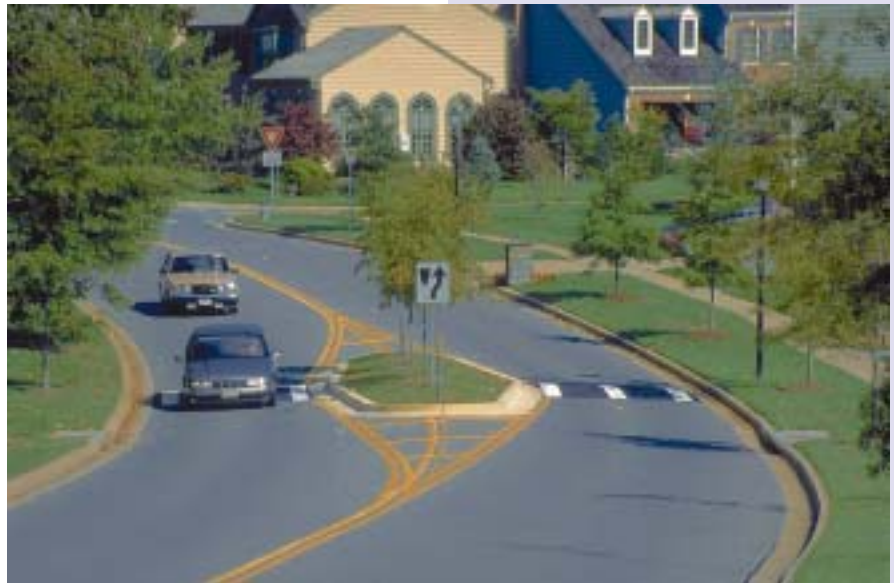
Speed hump with median island
